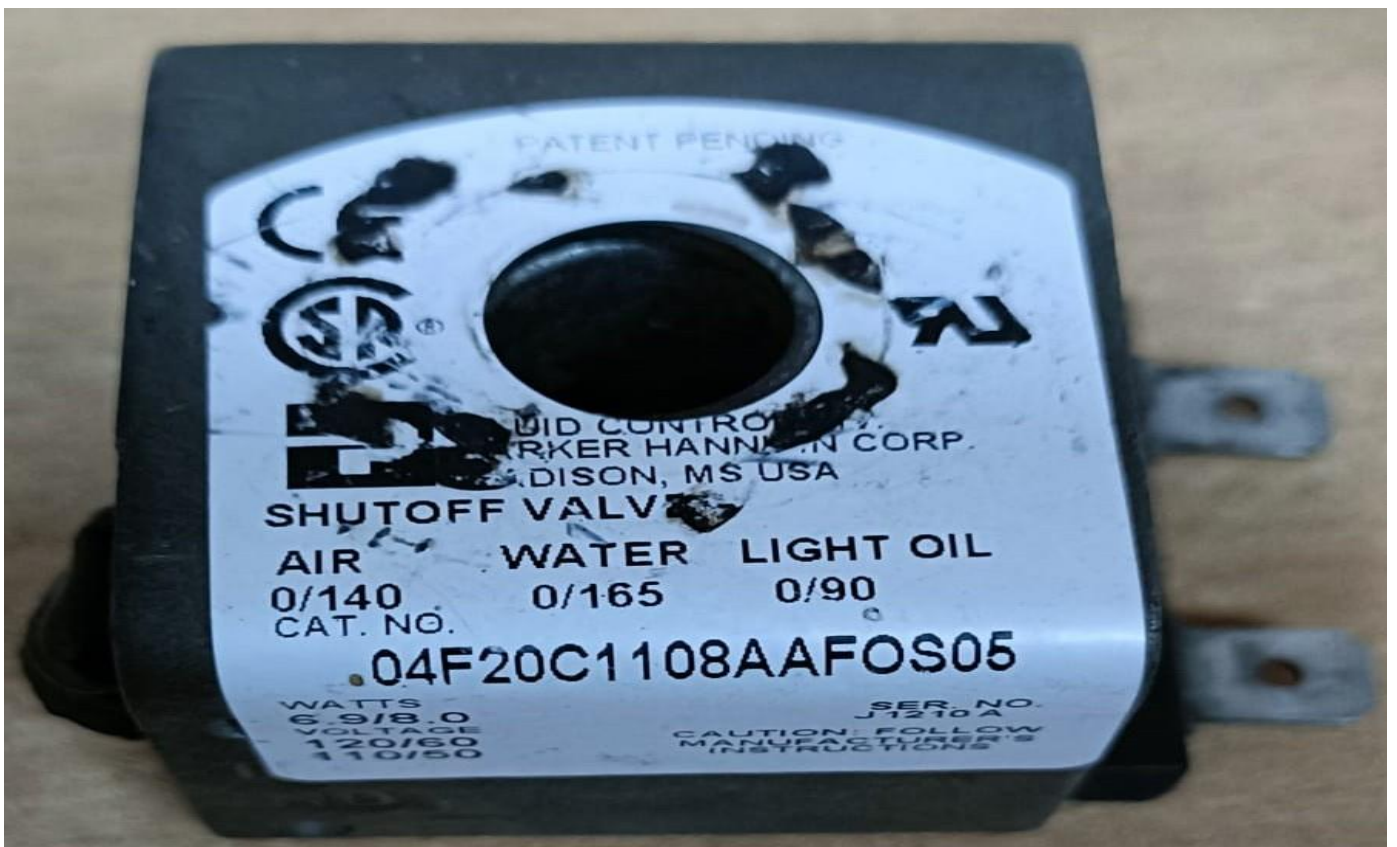
SHUT OFF VALVE
